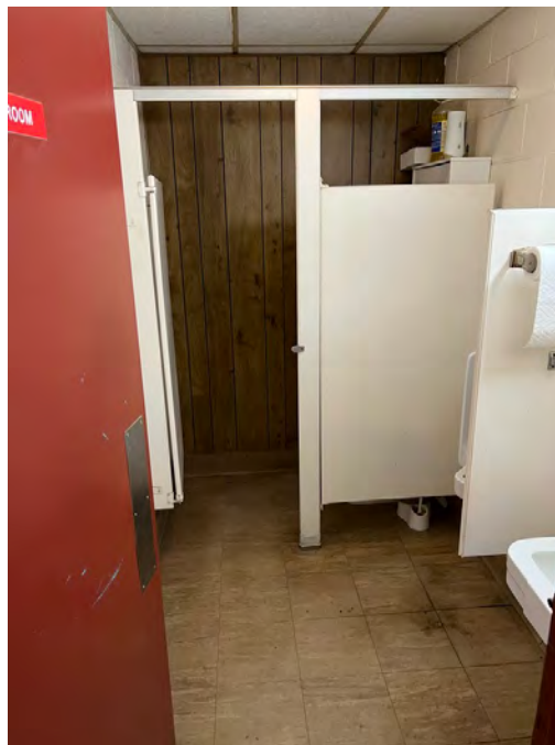
Photo 6 : Bathroom in Building One
