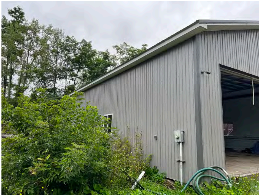
Photo 34 : Eastern exterior of Building Four
