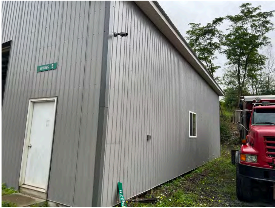
Photo 35 : Western exterior of Building Four
