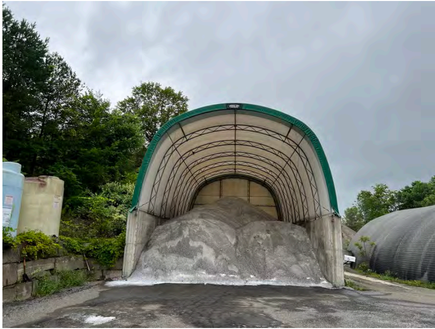
Photo 67 : Salt storage shed on northwestern portion of Subject Property
