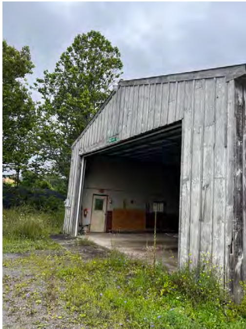
Photo 26 : Northwestern exterior of Building Three
