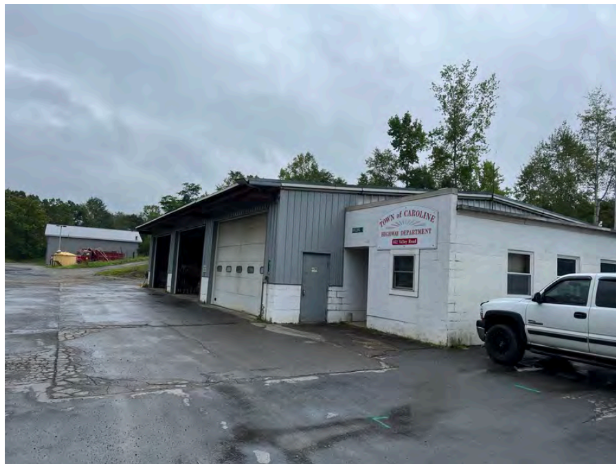
Photo 2 : Northern exterior of Building One
