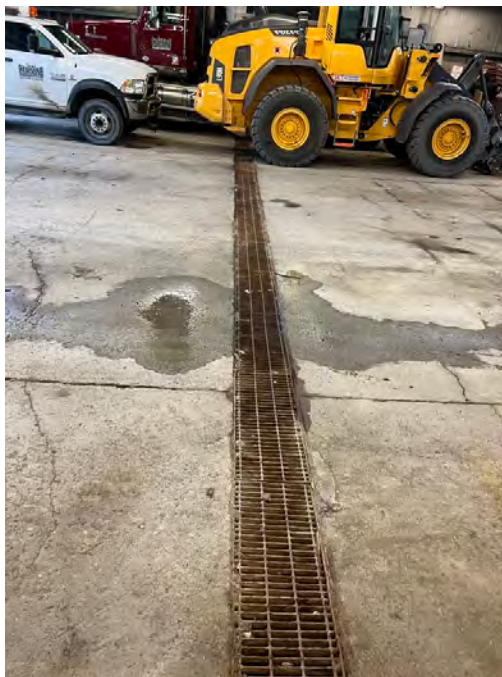
Photo 16 : Trench drain in garage of Building One
