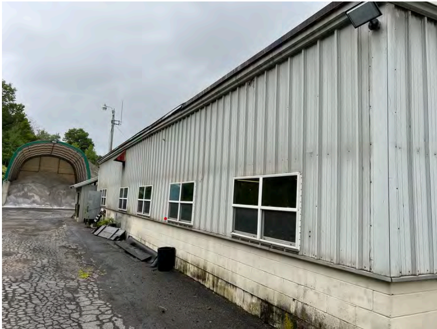
Photo 4 : Southern exterior of Building One
