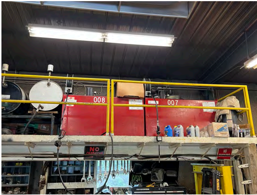
Photo 9 : 300-gallon motor oil and hydraulic oil ASTs in garage of Building One
