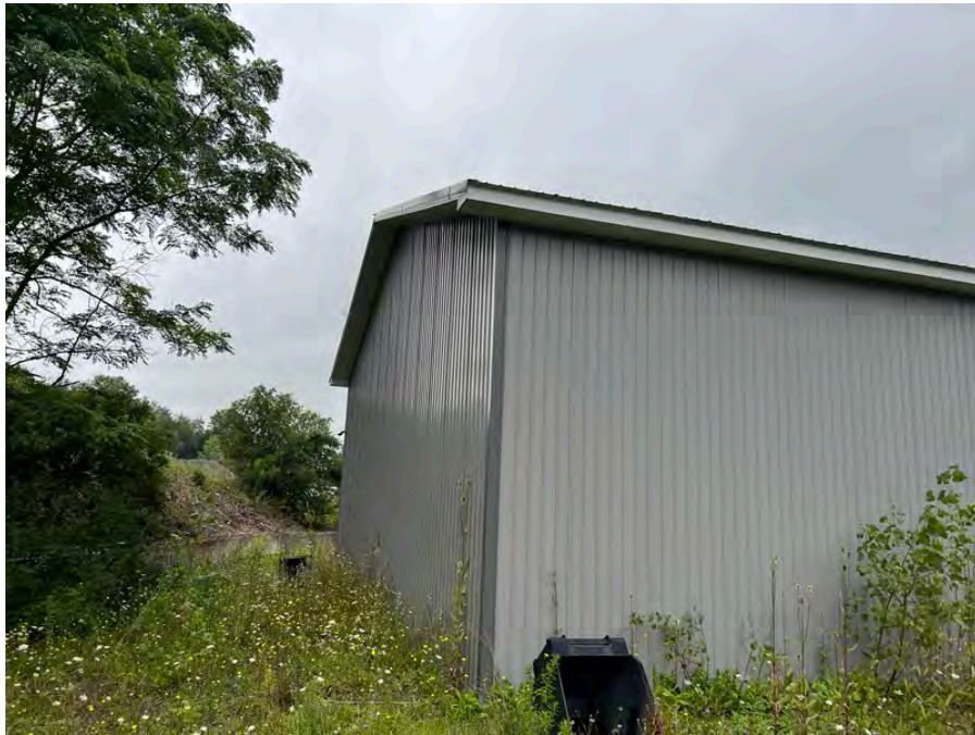
Photo 36 : Southern exterior of Building Four
