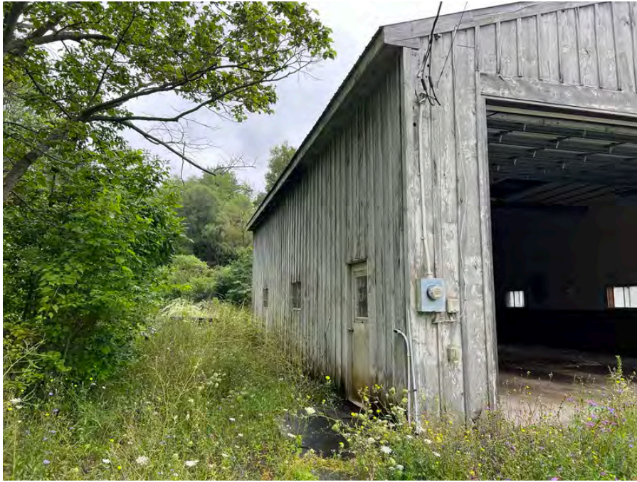
Photo 27 : Northeastern exterior of Building Three
