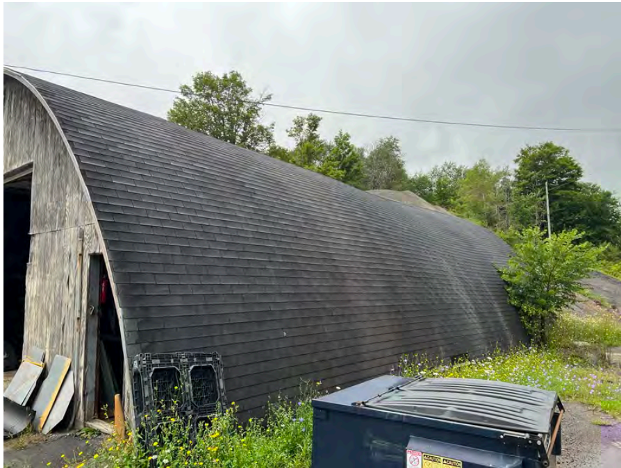
Photo 18 : Northern exterior of Building Two
