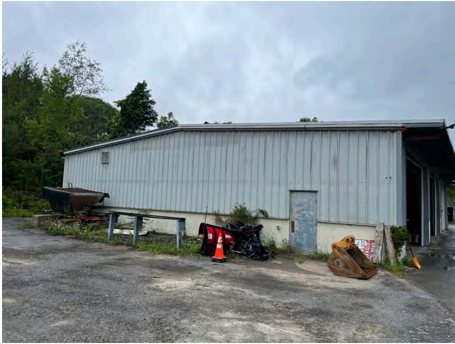
Photo 3 : Eastern exterior of Building One
