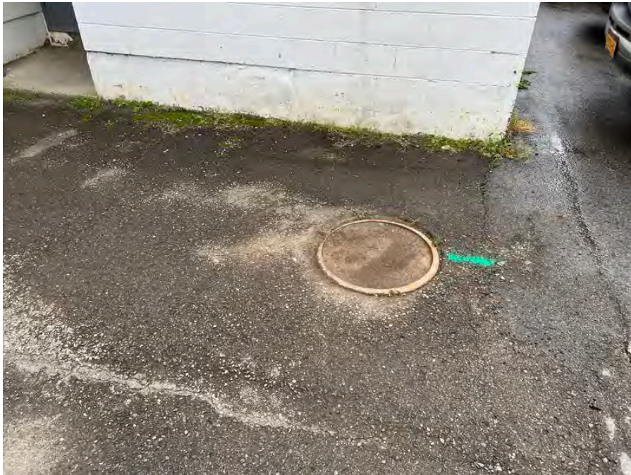
Photo 70 : Septic tank on northwestern exterior of Building One
