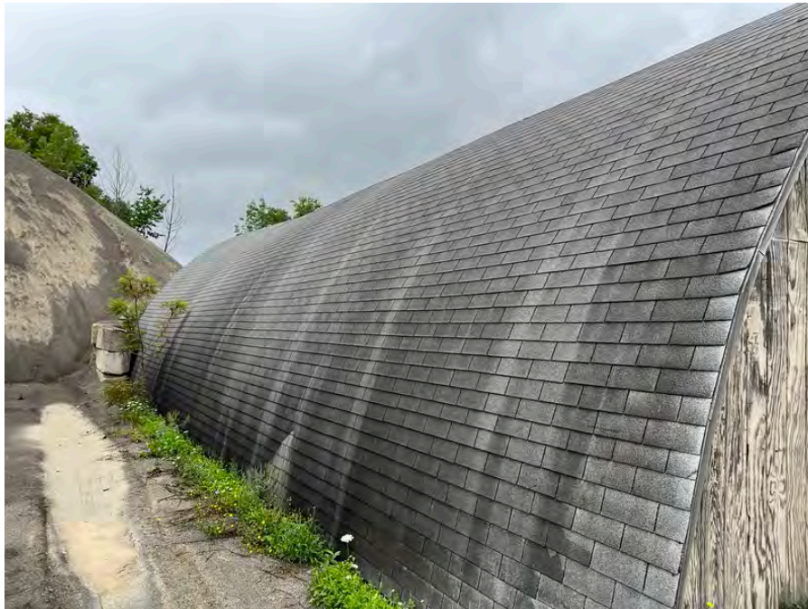
Photo 20 : Southern exterior of Building Two
