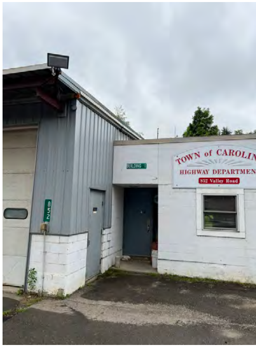
Photo 1 : Subject Property signage
