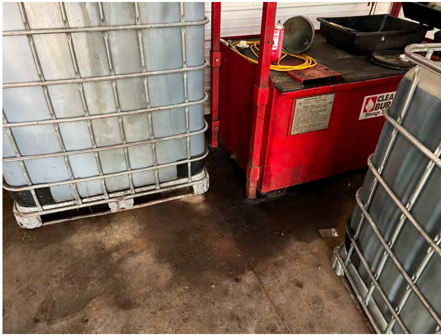
Photo 43 : Staining proximate AST in Building Four
