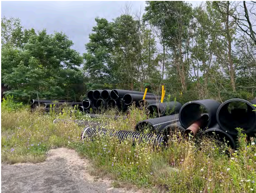
Photo 54 : Corrugated pipes on southern portion of Subject Property
