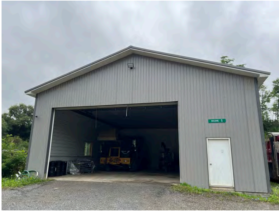
Photo 33 : Northern exterior of Building Four
