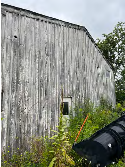
Photo 28 : Southeastern exterior of Building Three
