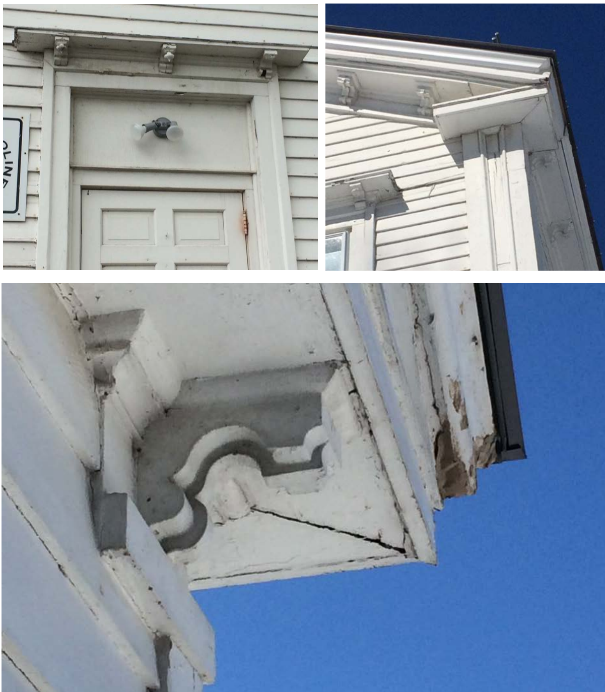
Figure 10. Ornamentation condition (Clockwise from top left) missing teardrop brackets, mild paint failure, and open joints and wood loss.
