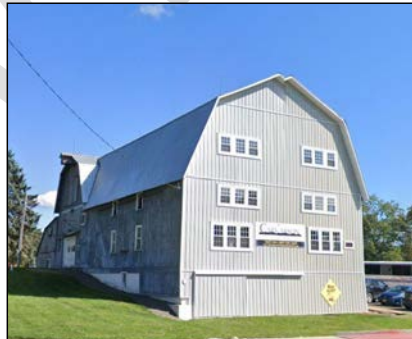
Carson Groundworks on Route 79
